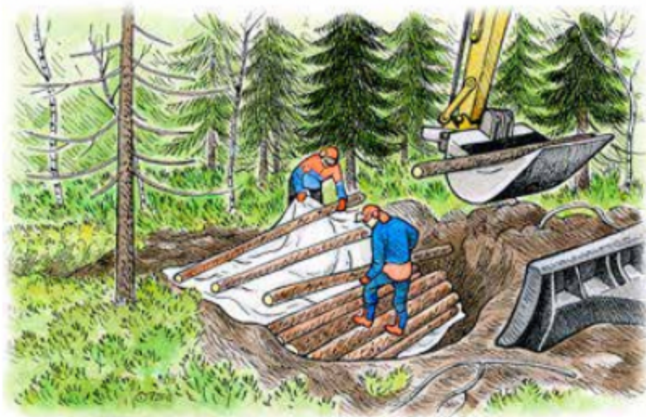
Figure 4. Example of wood dams to be built (from https://julkaisut.metsa.fi/wp-content/uploads/sites/2/2023/11/b188.pdf , p. 148).
